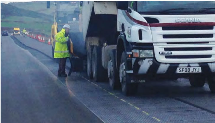
Tensor AR-GN can provide resistance to fatigue cracking and minimise fracturing due to long-term differential movements in the subgrade.
