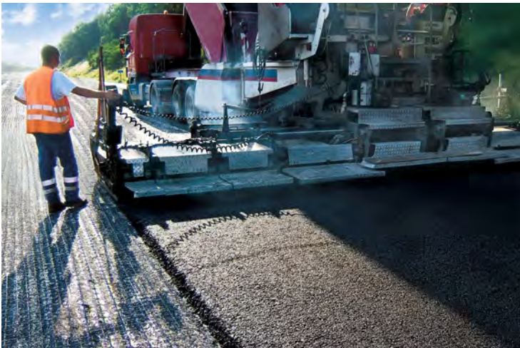
Paving takes place directly over the Tensor AR-GN
