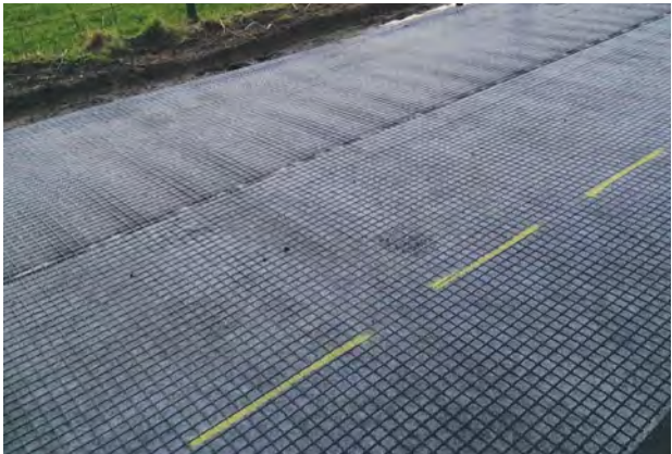
Tensor AR-GN can provide resistance to fatigue cracking and minimise fracturing due to long-term differential movements in the subgrade.
